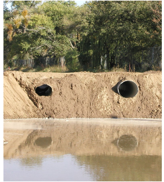
Canal seepage loss ponding test, Franklin Canal, El Paso, Texas
